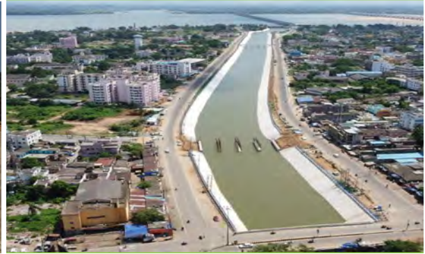
Taladanda Main Canal
