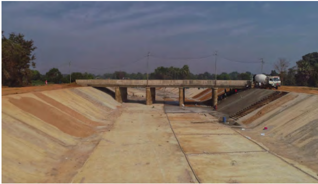
Lining of Baitarani Left Main canal (Anandapur Barrage)
